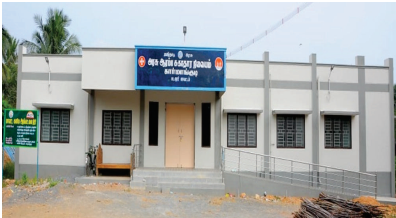
Construction of Primary Health Center at Karmangudi Village of Srimushnam Taluk in Cuddalore District at the cost of Rs.80 lakh
