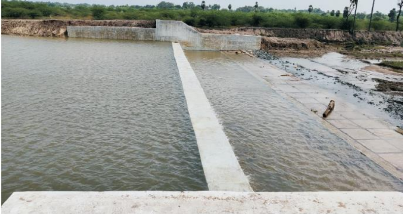
Check dam constructed across the Kallar odai in Kallankurichi village in Ariyalur district at a cost of Rs. 2 crore from DMFT Fund
