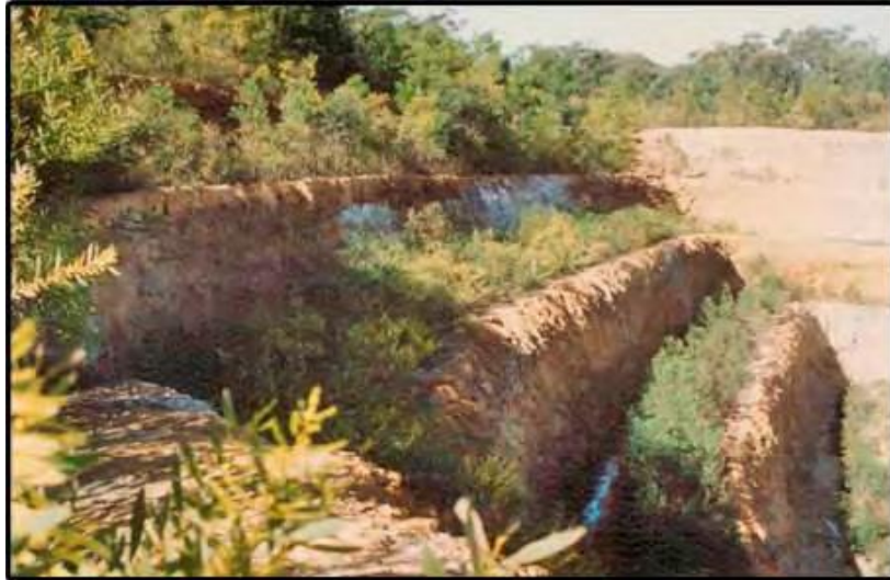
Figure 1: Example of Bench Rehabilitation
