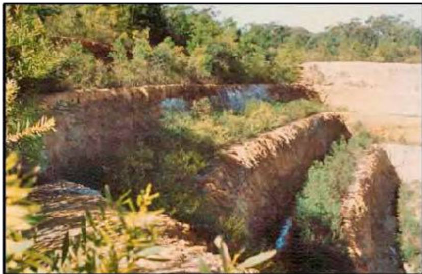
Plate 9- Example of Bench Rehabilitation
