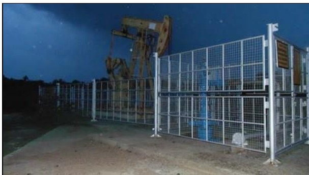
Sucken Rod Pump mechanized flow well near Vijayapuram # 13 area, Thiruvarur (Location: 10°45'43.32"N 79°38'30.32"E)
