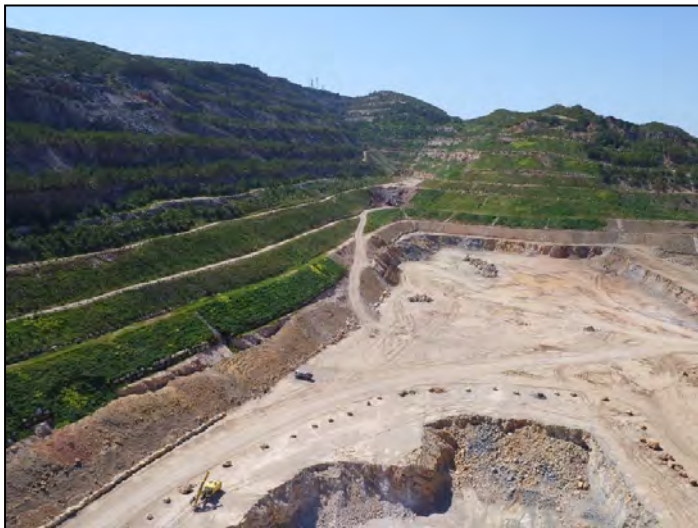
Figure 1: Example of Bench Rehabilitation
